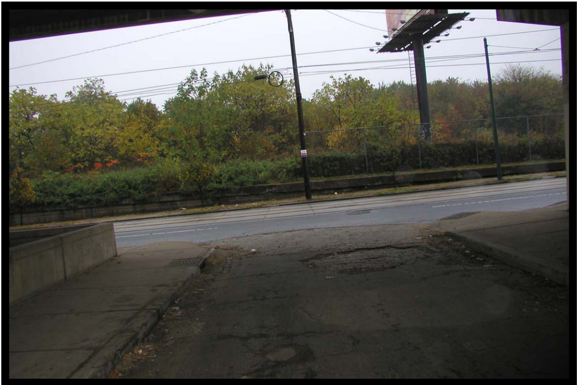
Plate 7.6 Sergeant Street, East of I-95, Facing East.
