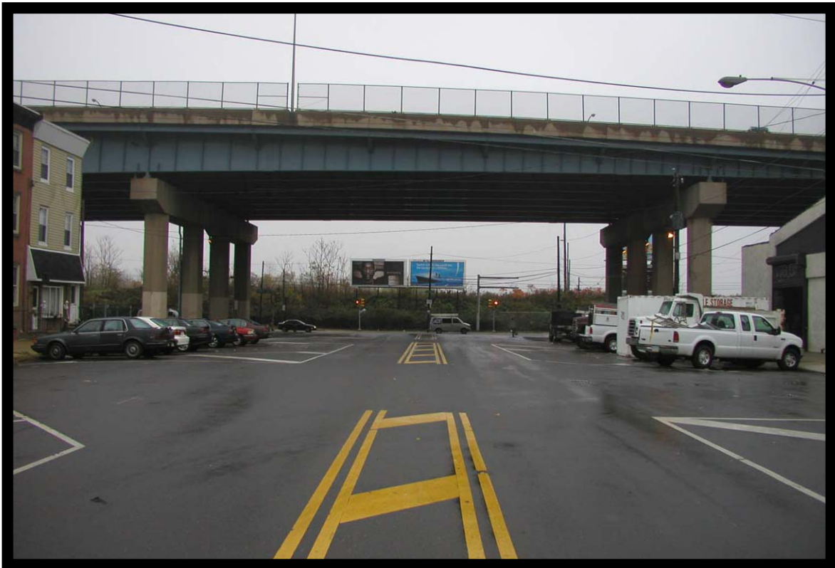
Plate 7.10 Lehigh Avenue, West of I-95.
