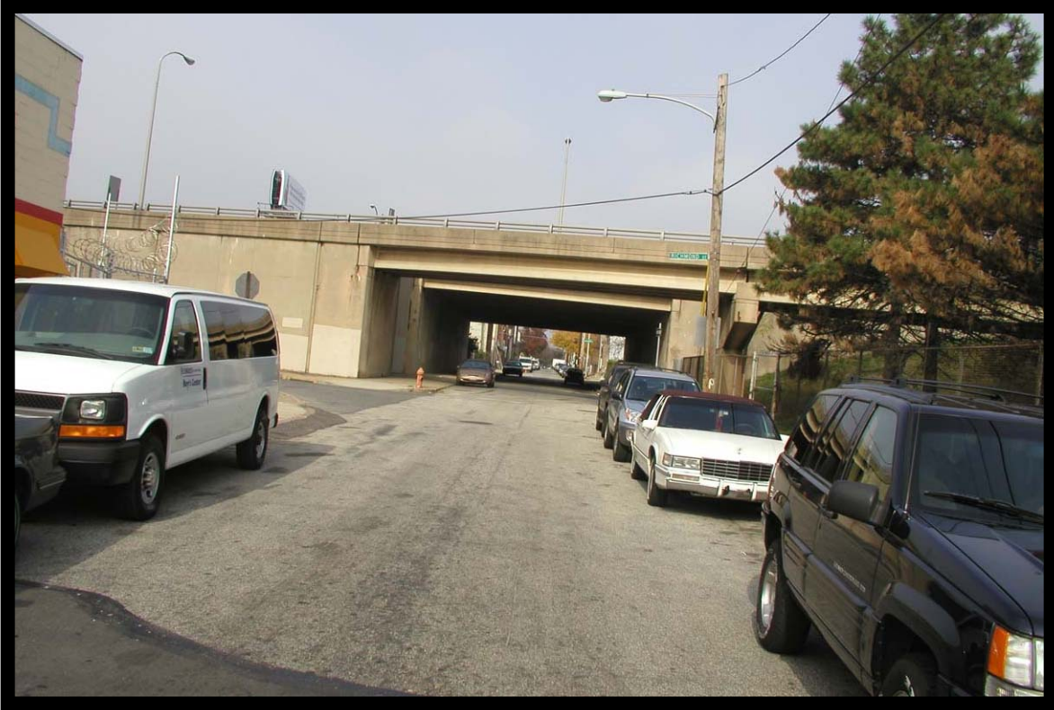
Plate 5.3 Columbia Avenue, East of I-95.
