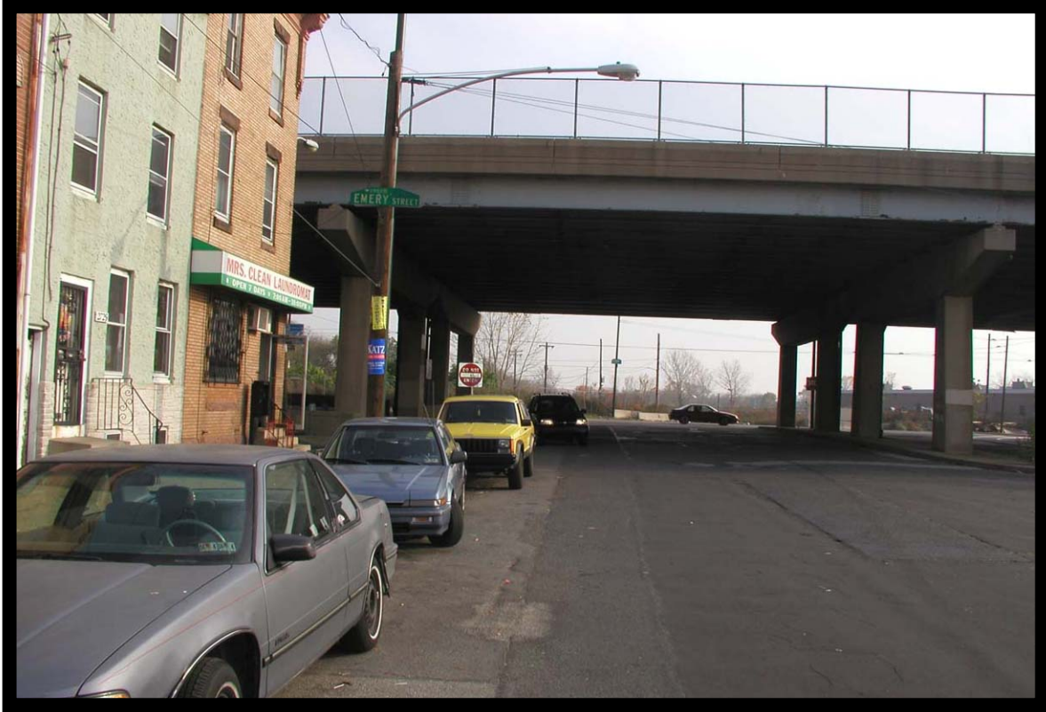
Plate 7.5 Cumberland Street, West of I-95.
