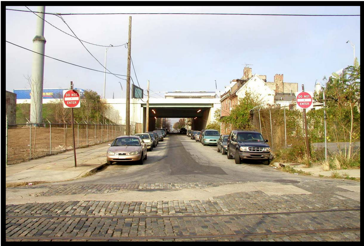
Plate 2.7 Brown Street, East of I-95.
