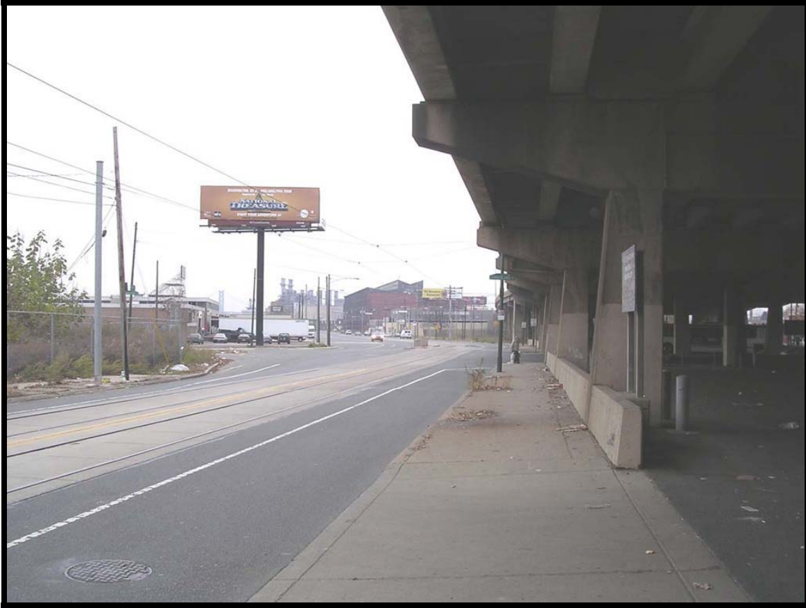
Plate 8.1 Intersection of Cumberland Street and Richmond Street Looking South.
