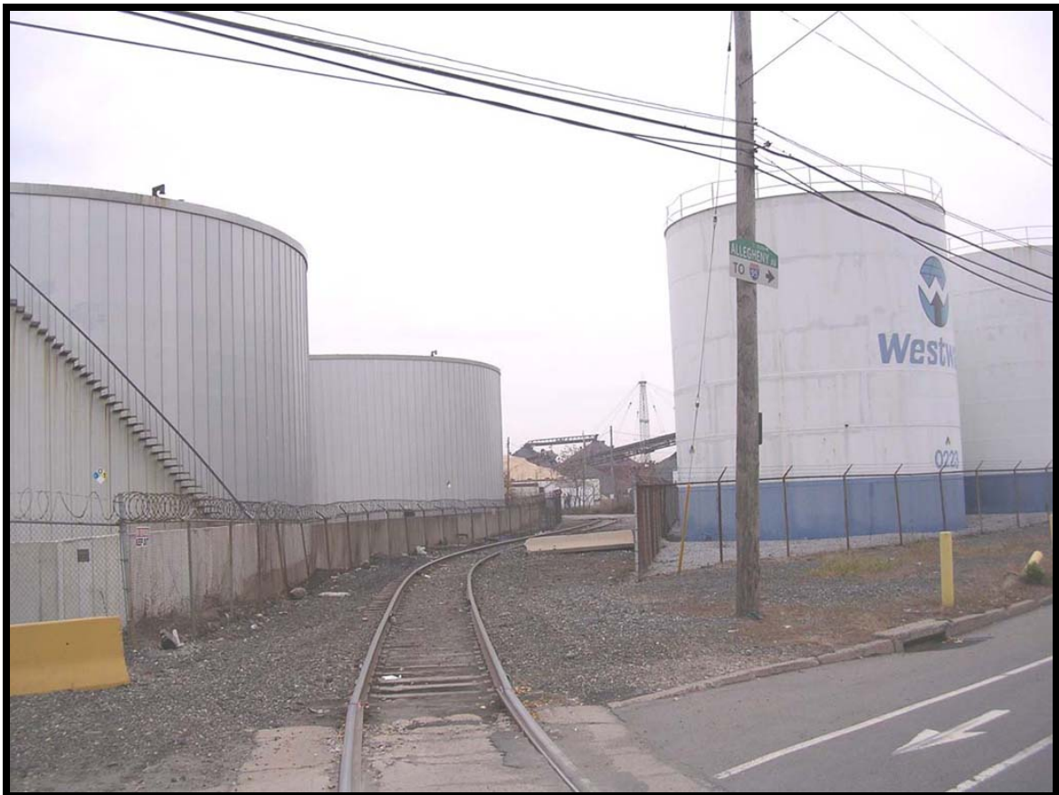
Plate 9.2 Tanks on Allegheny Avenue Looking South.
